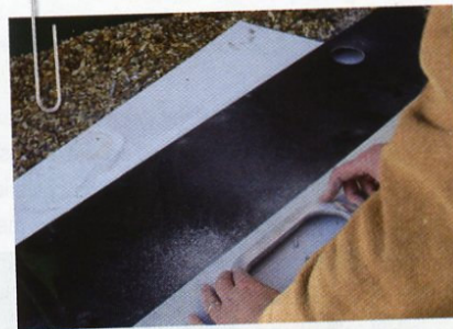
Final fettling using the polished aluminium surround as a template.
