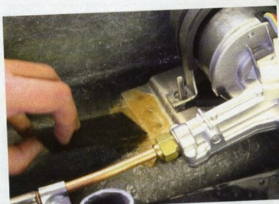
Bonding wiper motor bracket in place.
